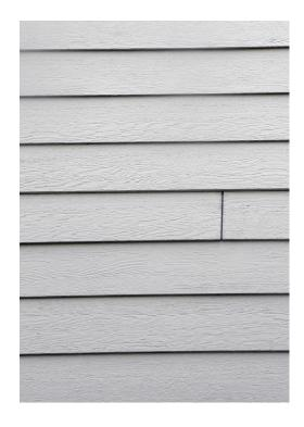
Joints must be properly maintained to prevent water penetration. The required 3/16 in. gaps at butt joints need caulk or clips, which increasingly accentuate the gaps since they can fade at a different rate than the siding.
